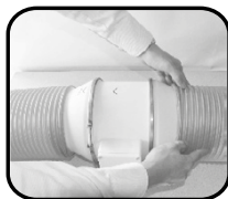
6. Connect the ventilation ducts
