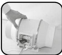
5. Make the electrical connections
